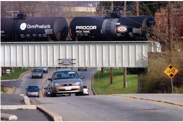
Harrisburg Pike under this railroad bridge would be widened to four lanes as part of proposed roadwork for “The Crossings” shopping center.
